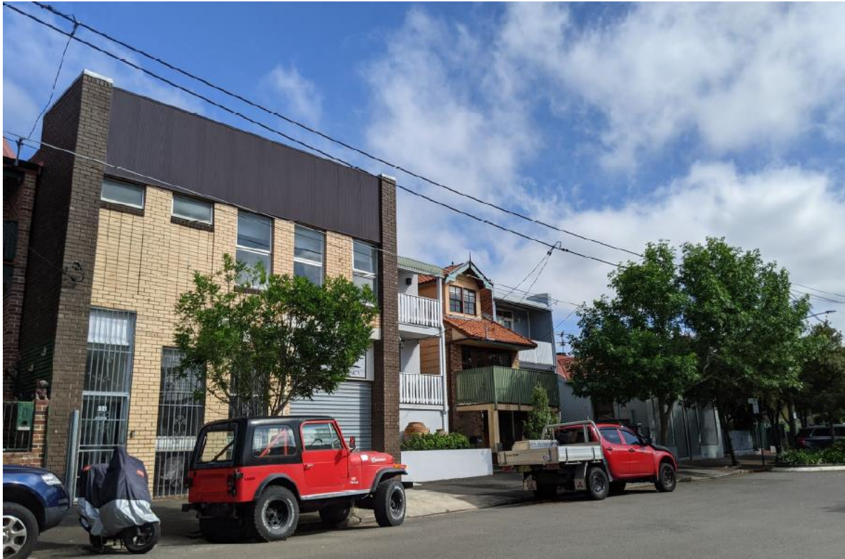
Figure 7: Commercial building at 124-126 Victoria Street and two storey terraces at 118-122 Victoria Street
