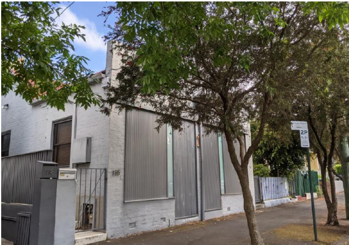
Figure 6: Pair of single-storey terraces (114-116 Victoria Street) viewed from Victoria Street
