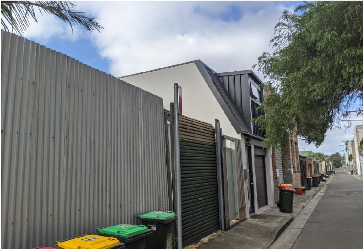
Figure 9: Existing laneway structure at the rear of 122 Victoria Street
